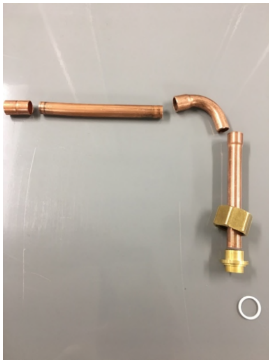
7. Separate pieces – braze pieces with Teflon Gasket removed... FLOW NITROGEN while brazing.
